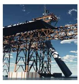
The erection of the first tower sections marks a new direction for SAS construction – straight up. From tipping up the 2.3-million-pound tower leg sections to building the erection tower and tower crane, vertical construction adds a new dimension to the already astonishing and unprecedented engineering and construction that is synonymous with the seismic retrofit of the Bay Bridge.
